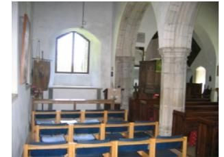
The North Aisle was added in 1350, the Arcade and pillars being of Caen stone, from France and brought up the River Chelmer to Sandford Mill, and then by cart to Sandon. The wall plate where the aisle roof joins the roof, was originally much lower as the bulge in the wall shows, indicating a rather low roof. The roof was renewed in 1878 in fir.
